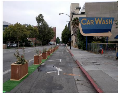
Wooden planter boxes as barriers along bikeway
