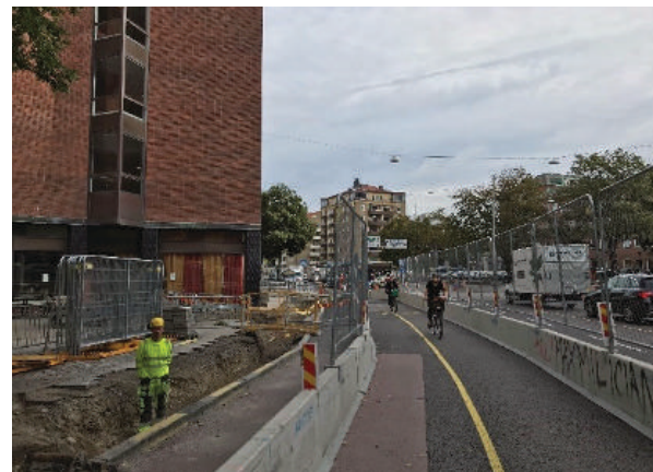
Figure 4.22 (a) Rerouting facility [70] .
